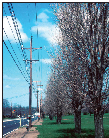
Tall, upright trees can be planted along, but never under, overhead lines.
