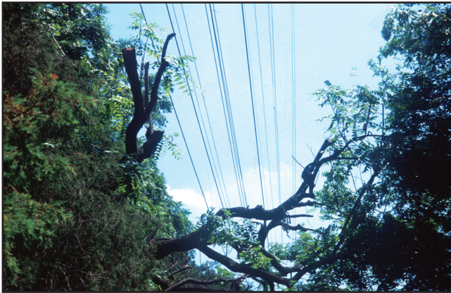
Directional pruning for line clearance.
